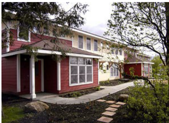
Douglas Meadows incorporates green building techniques into a small affordable housing project. Human Solutions sponsored this eight unit building with large apartments affordable to households earning no more than 50% of area median income, with two apartments set aside for extremely low income families.
